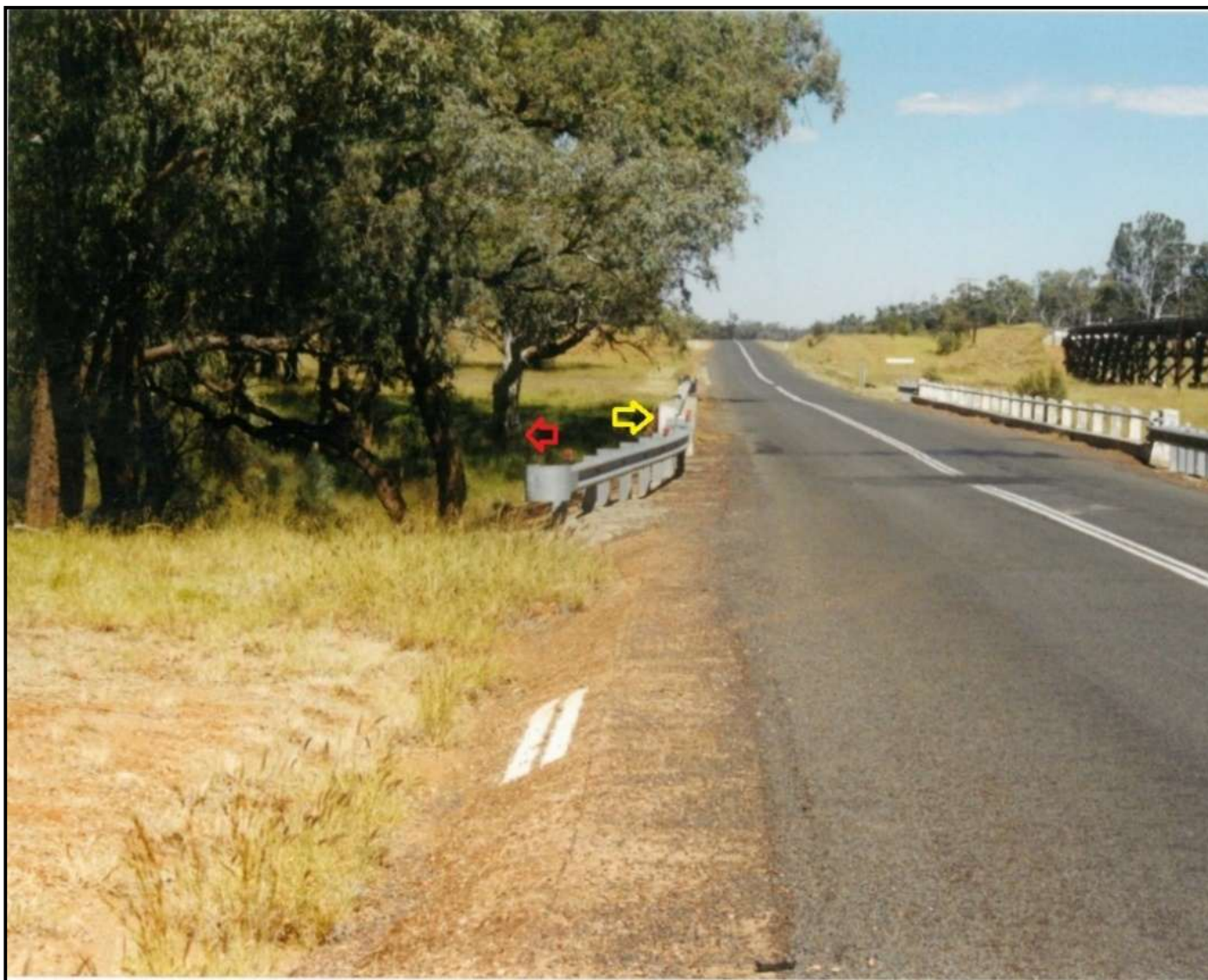
Picture 1 – Angellala Creek Bridge prior to incident
