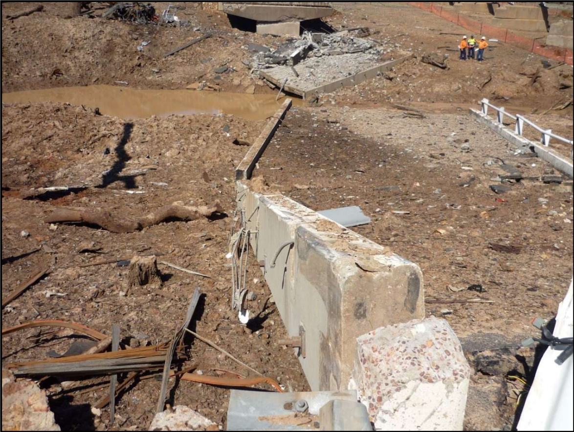
Picture 5 - Parapets show black marks and the bent rail brackets
