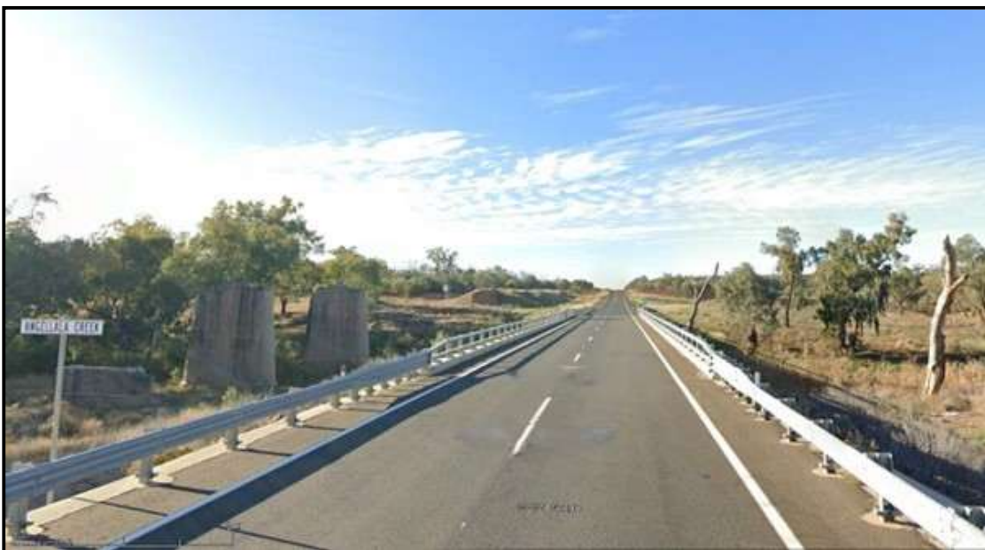
Picture 24 – Heroes Bridge at Angellala Creek heading north
