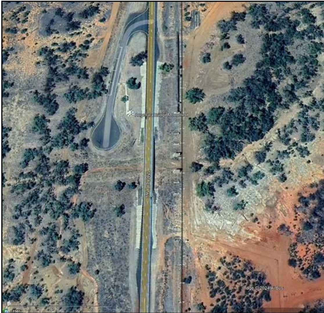
Picture 25 – Overhead of Angellala Creek Bridge and monument site
