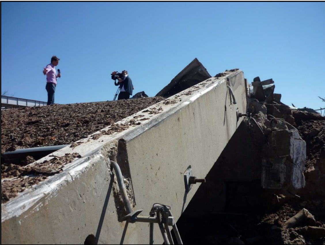
Picture 5 - Parapets show black marks and the bent rail brackets
