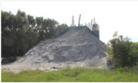
Above and Below: Preparation of building to withstand blast and direct sound away from community
