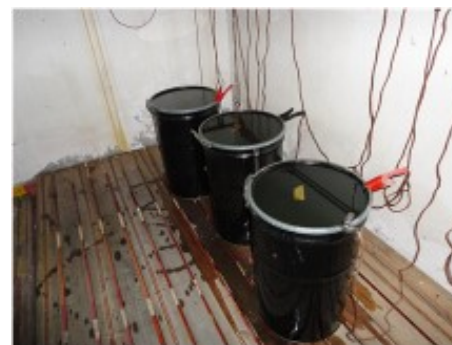
Tetrazene oozing out of drums running down on side and underneath drums due to pit corrosion.
