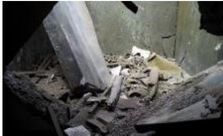
Above: Lead styphnate coloration in one corner of building after the blast.
