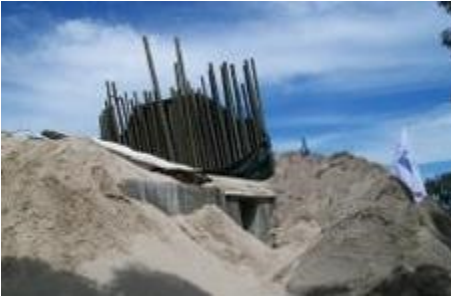
Above and Below: Preparation of building to withstand blast and direct sound away from community
