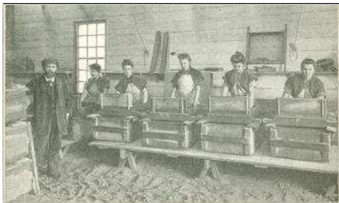
Interior of a mixing house
