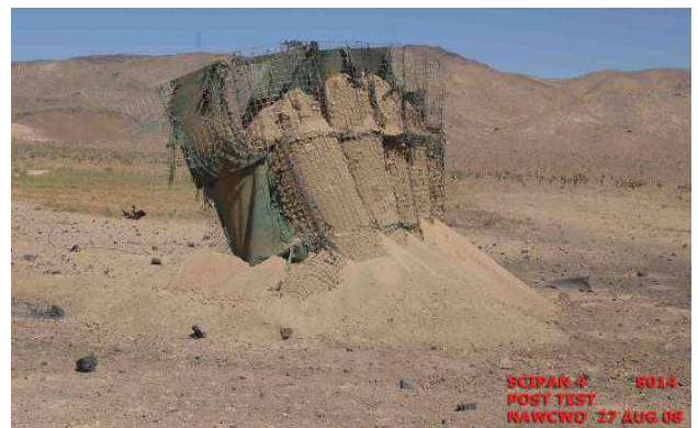
Figure 5: Barricade Remains—Post Detonation
