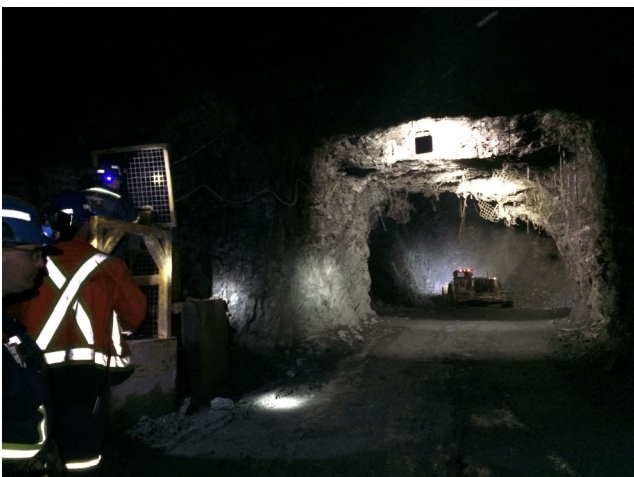
Remote mucking at the undercut level
