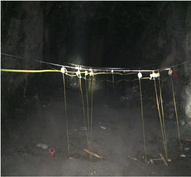
Loaded holes at the overcut level
