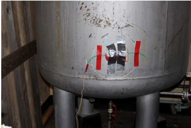
Figure 21 – Explosive charge on vessel
