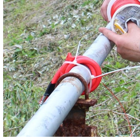
Figure 25 and Figure 26 – Detonating cord applied on steel pipes
