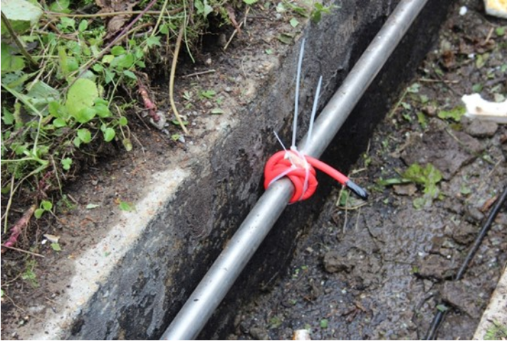
Figure 25 and Figure 26 – Detonating cord applied on steel pipes
