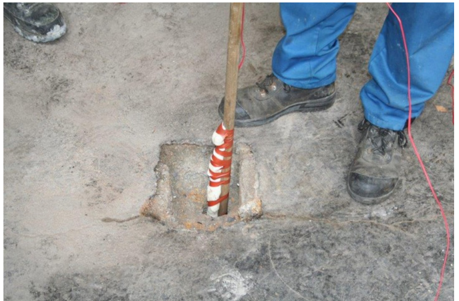
Figure 14 – Stick with explosive charge
