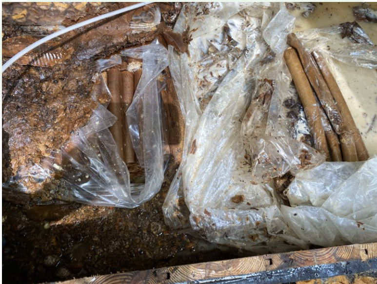
Dynamite Soaked with MuniRem Solution to Allow for Safe Recovery
