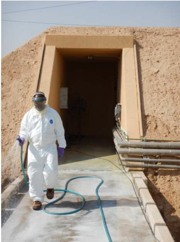
Spray Application of Chemical Neutralant to Render Safe Entrance into Explosives Storage Magazine
