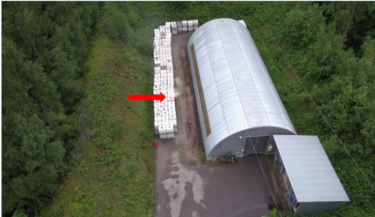
Figure 1. Storage building 312 (ANFO storage) and the placement of the IBCs – the IBC generating steam is marked with an arrow.
