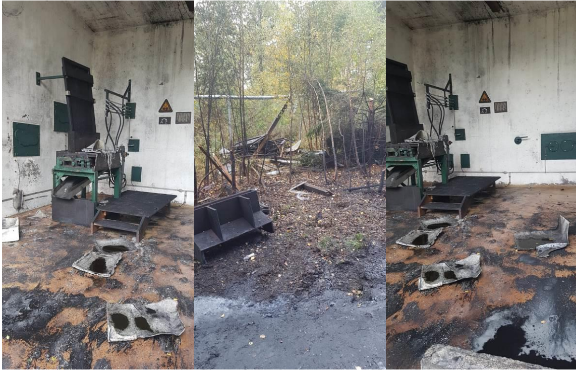
Building 55/2 after the accident
