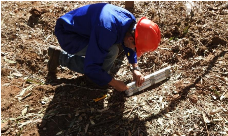
Figure 11: Placing of Charge
