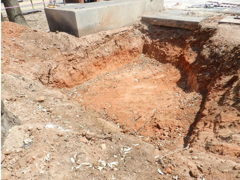
Figure 17: Single hole after cleaning
