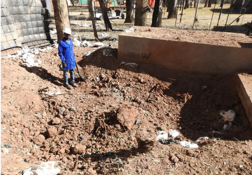
Figure 14: Final crater after last blast
