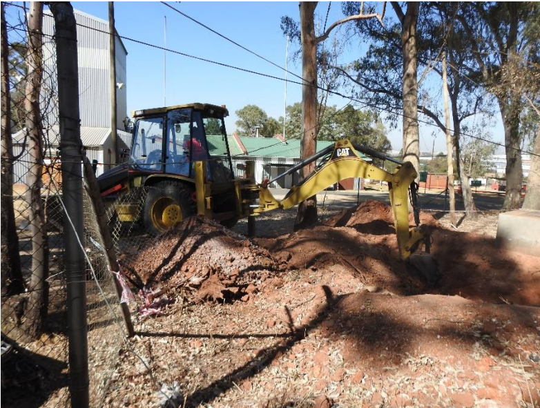
Figure 16: TLB clearing crater of loose material
