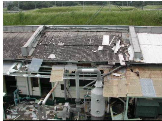
Photo.4 Outside view of the granulating and drying room
