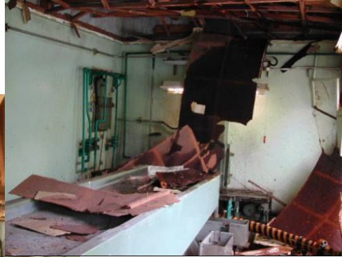
□ d dry conveyor and ceiling
