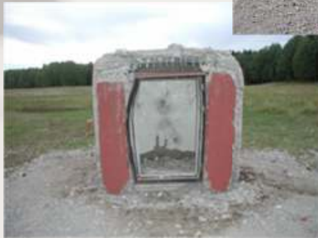
Vented (door removed)
