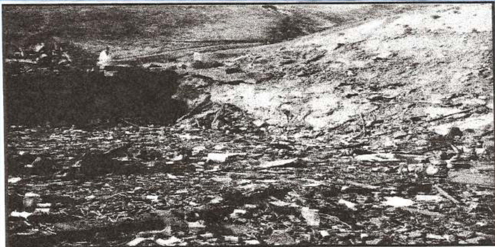
Figure 8. Booster Room 2 After Explosion
