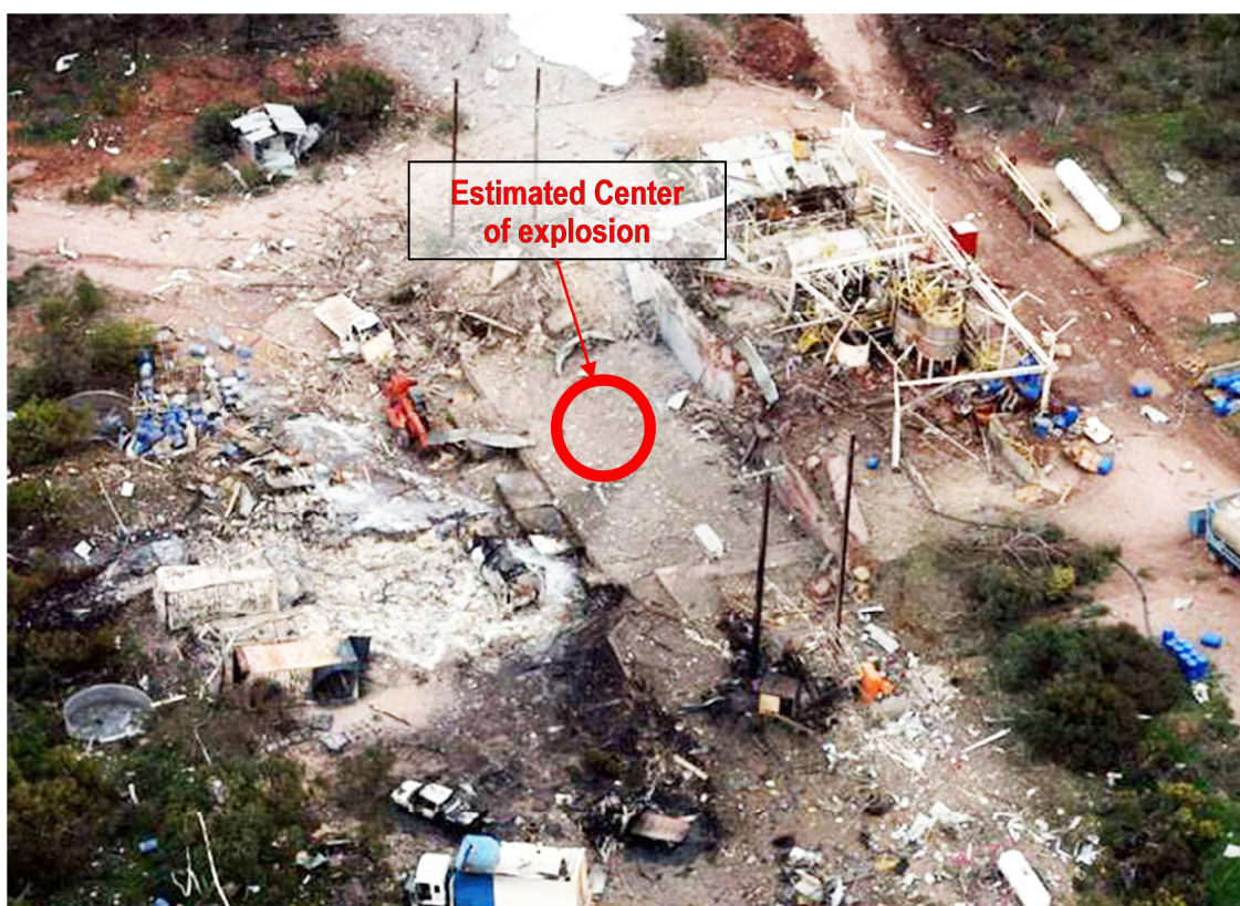
Figure 8. Quin Site Accident
