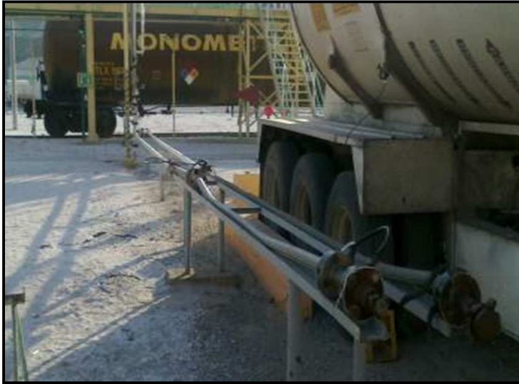
Picture 1: MMA unloading area with tanks and unconnected discharge hoses
