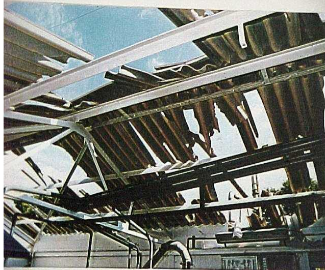
ROOF OF BUILDING 50M AWAY
