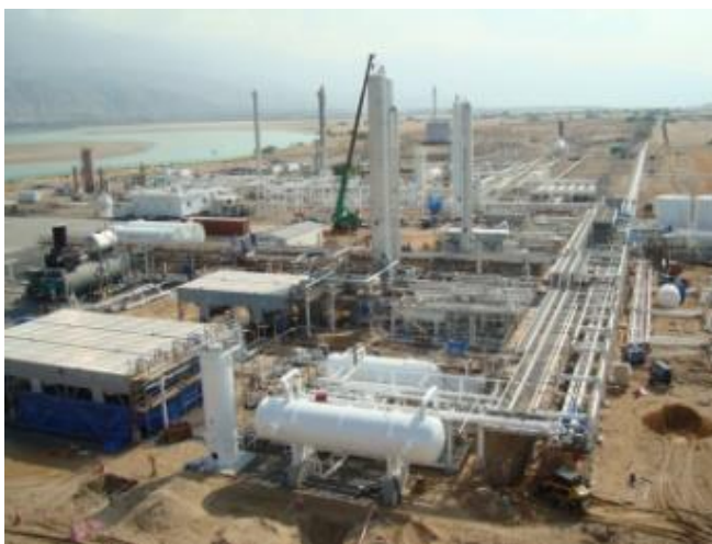
Figure1: Installation of the new processing train
