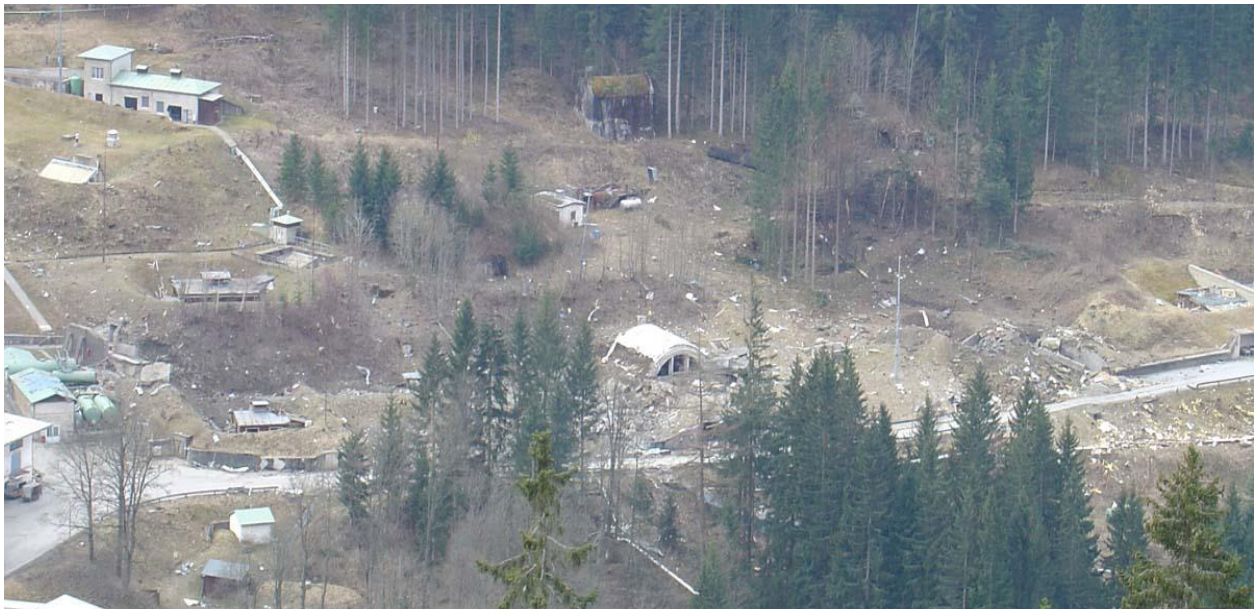
Figure 2 - Mixing house after the accident
