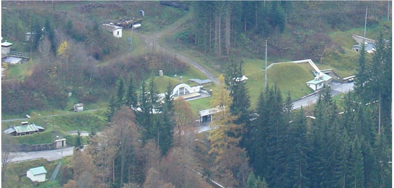
Figure 1 - Mixing house before the accident
